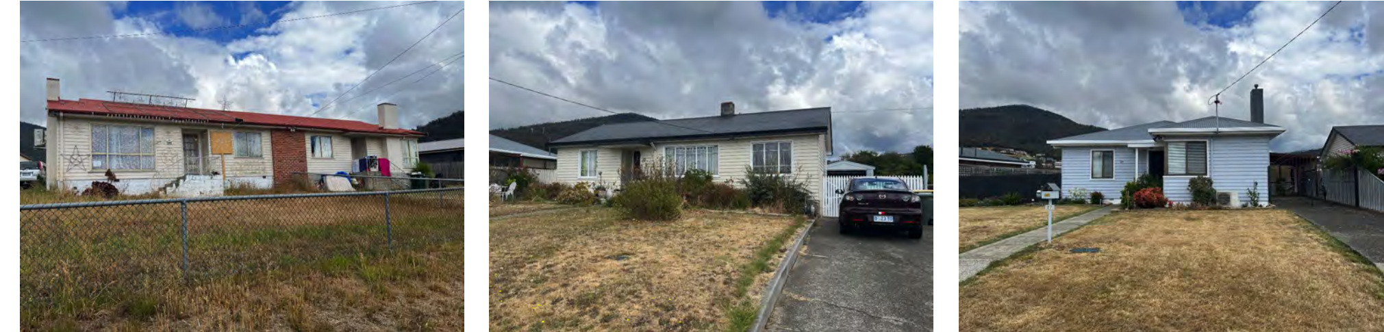
SINGLE STOREY WEATHERBOARD COTTAGES GABLE + HIP ROOFS
